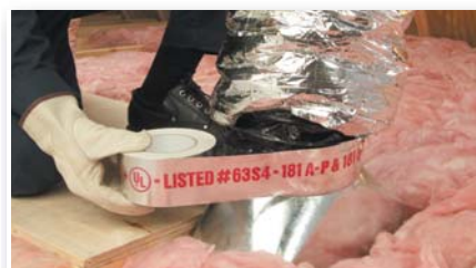
To seal fiberglass duct board and flexible duct systems, Scotch® Foil Tape 3326 meets the performance requirements for UL 181A-P and UL 181B-FX. 317
